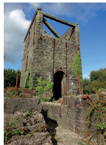
Bailey's Shaft engine house, Hingston Down Mine
