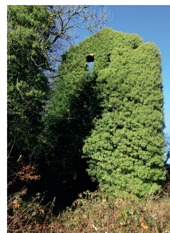
Ivy-covered remains of Hitchen's pumping engine house
