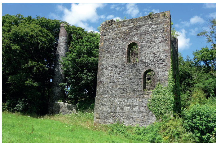
Chimney and winding engine house, Holmbush Mine: remnants of a once-flourishing industry
