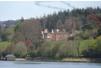
Maristow House, with the quay below
