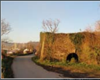
(Left) A pair of back-to-back late 18th / early 19th century rubble stone limekilns at Weir Quay.
