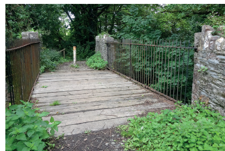
Bridge over the inclined plane
