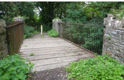
Bridge over the inclined plane
