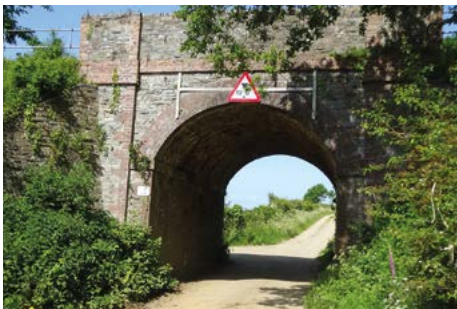
The route passes under the Tamar Valley Line railway bridge
