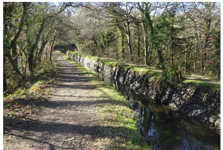
An aqueduct carries the canal across the valley of the River Lumburn
