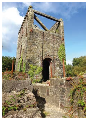
Hingston Down Mine engine house
