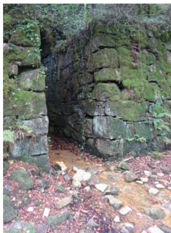
The waterwheel pit, Riverside engine house, Gunnislake Clitters Mine
